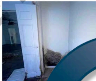
Mold-like growth flooring and dryw
