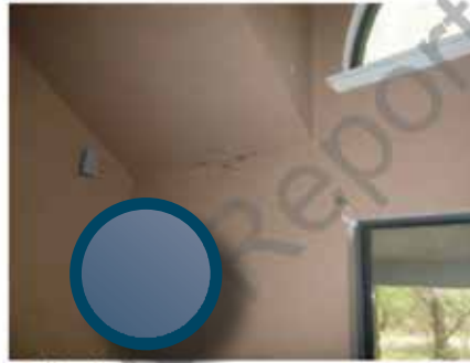
Wall and ceiling
