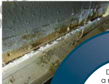
Baseboard and lower wall
