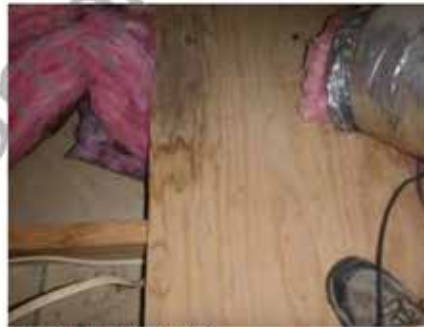
Decking at HVAC unit
