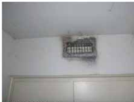
Wall at HVAC supply
