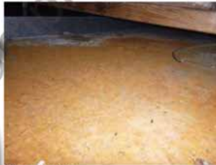
Rusty drain pan
