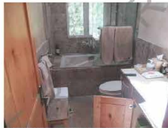
The client reported that the water loss that affected the Basement SE Room originated from the tub area while it was in use.
